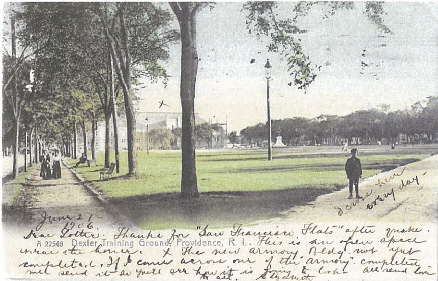
The Armory under construction. The text, written in 1906, reads: "I cross here every day."
